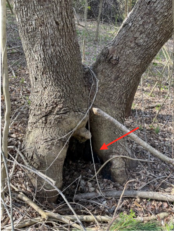
Tree 600 - Resprout from stem failure; Cavity in base
